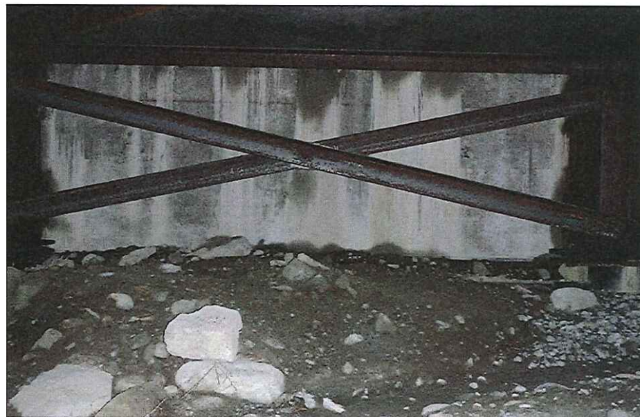
CK2099 Abutment Left Bank
