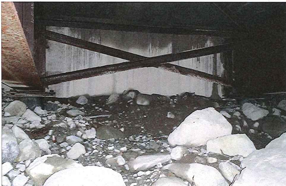
CK2099 Abutment Right Bank
