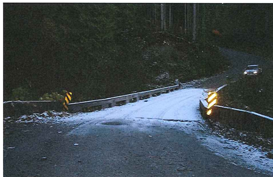
CK2099 Approach Right Bank
